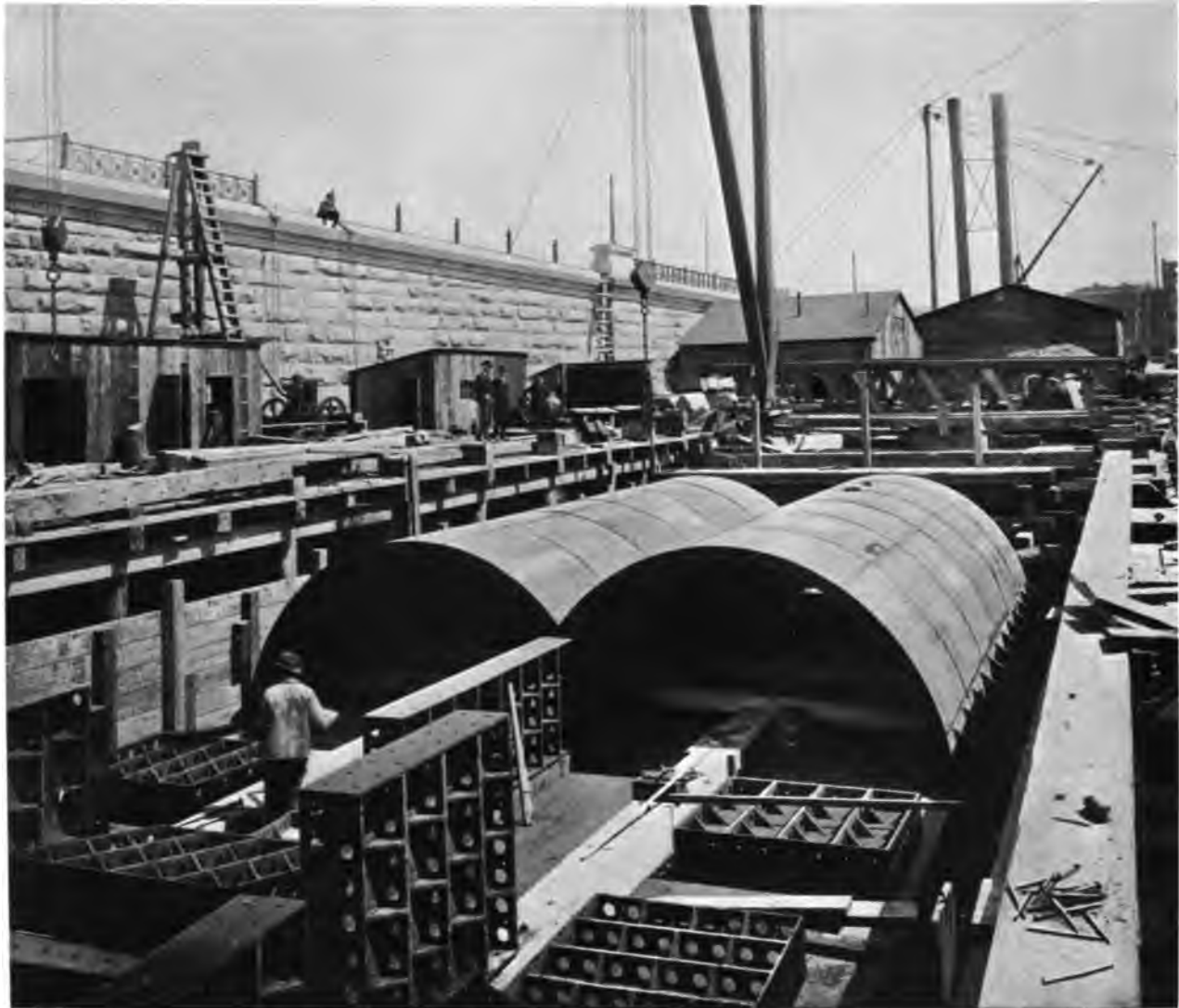
ASSEMBLING IRON WORK ON PONTON — HARLEM RIVER TUNNEL
